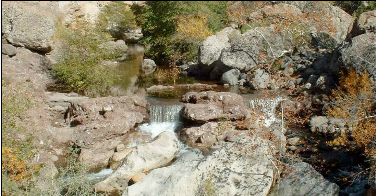
Figure 13. Fossil Creek Fish Barrier as constructed.
