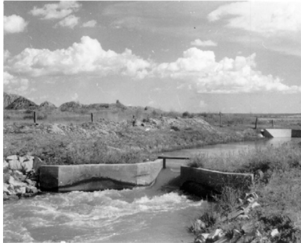
Four-foot short Parshall flume, discharging 62 cfs under free-flow conditions; scour protection is needed for this much drop. Photo from: USBR Water Measurement Manual – Chapter 8.
