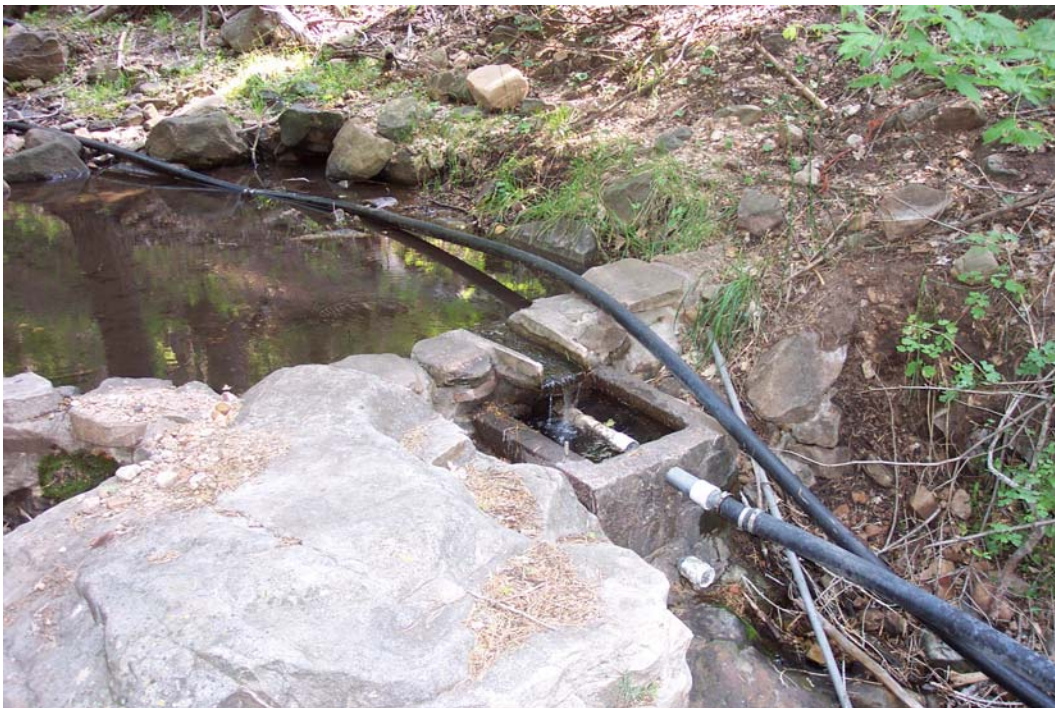
Figure 21 – Dam in spring channel and pipes diverting flow for private use (Washington Spring 8/12/02).
