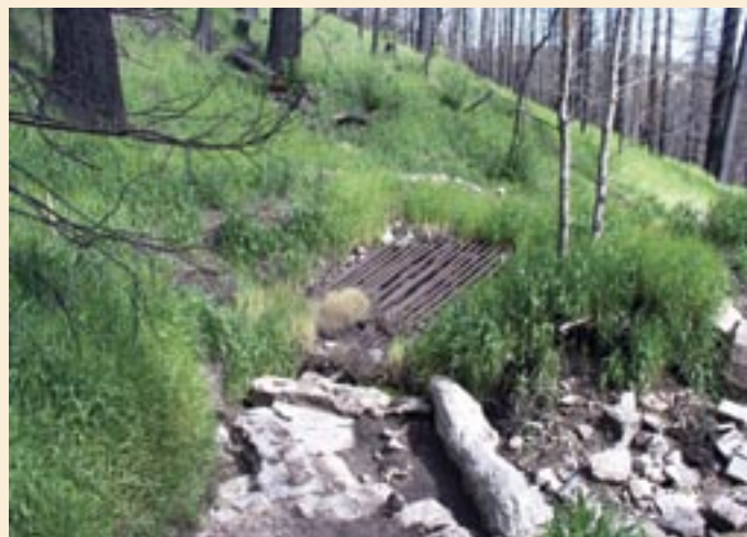
Trash rack constructed to prevent large debris from washing downstream in Carter Canyon, Santa Catalina Mountains, Arizona. Top: July 17, 2003, just after containment of the Aspen Fire. Bottom: Oct. 12, 2003, showing three months of regrowth. Photos from the Aspen BAER Treatment Monitoring Report, Appendix B.
